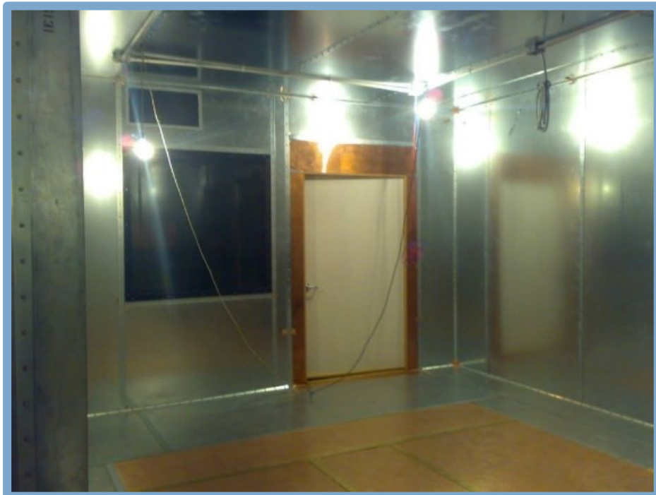
RF shielding construction technique implemented in one of our projects.
